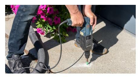
Vacuum (or blow) the drilling dust and debris to leave a clean hole. A screwdriver can be useful to loosen any debris in the hole.
