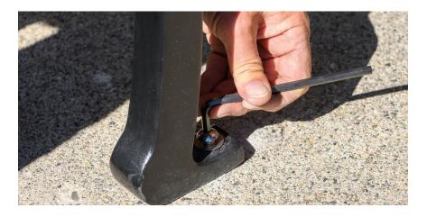
Optional. For theft resistance, fill in the bolt heads with silicone and paint the tops of the fasteners with a paint pen to match the colour of the frame.
