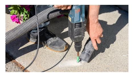
Hammer the concrete anchors into the clean drilled holes so they are slightly below flush with the surface. This is easiest with a sacrificial bolt.
