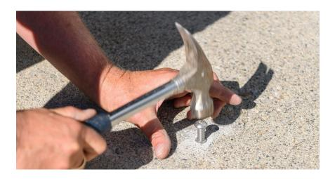
Fix the anchors in place with the supplied set tool and a hammer to expand the base of the anchors and permanently secure them to the pad.
